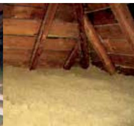
Blown-on process for open, horizontal structures
