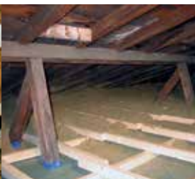
Blown-on process for open, horizontal structures
