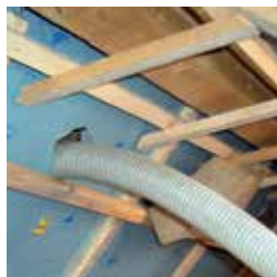
Roofing: our insulation is blown into the existing structure
